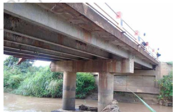
Figure 5: Bridge underside showing steel beams and pier.
