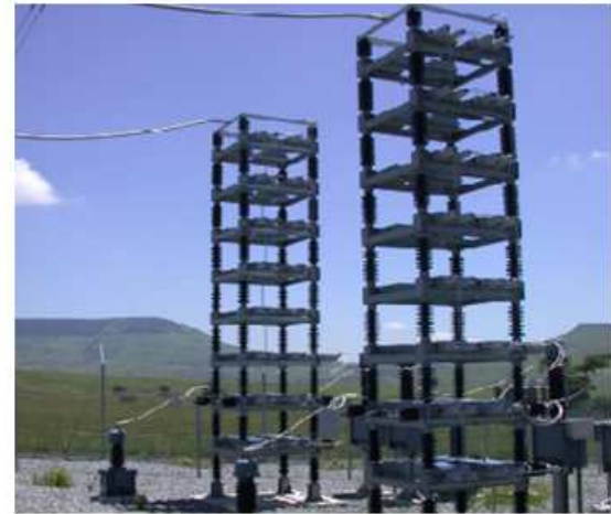
Figure 1. (a) and (b) Single line and pictorial diagram of a CCS
